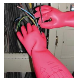
Figure A3.3.2c.7: Insulating gloves Protection class 00 (500V) Protection class 0 (1000 V) Protection class 1 (7500V) Protection class 2 (17000V) Protection class 3 (26500V)
