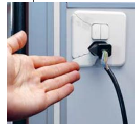
Figure R4.1.7.5: Example of defective barrier and plug
